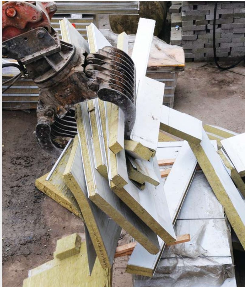
Mobile recycling unit shredding composite panels.
